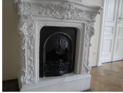
The fire place in the upper hall. The door to the small classroom is on its right
